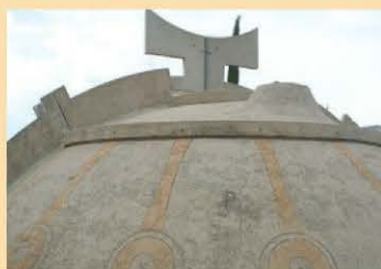
Soleri's concrete half-domes are built into the earth.
